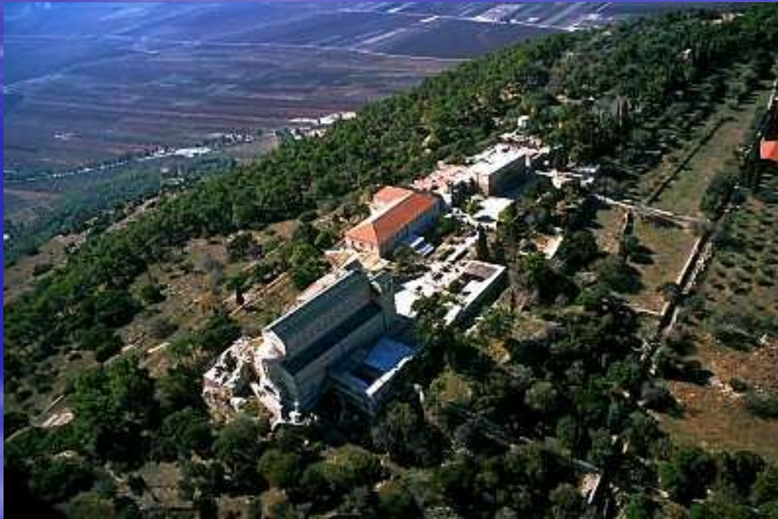
Aerial view of the Church of the Transfiguration on the summit of Mount Tabor
